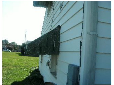
left side of exterior
