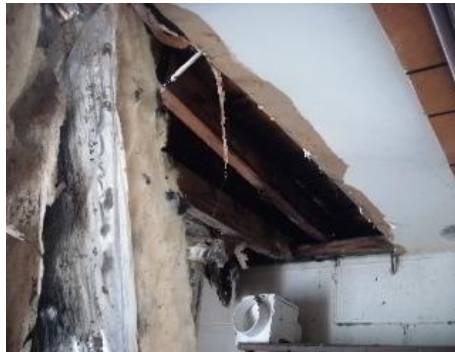
ceiling in laundry area
