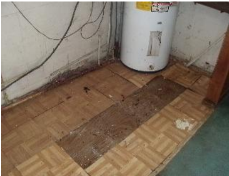
laundry area and floor
